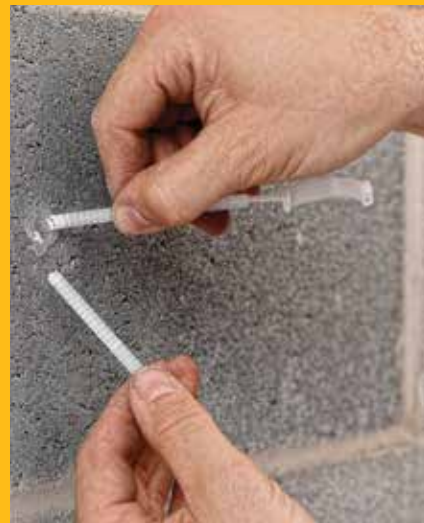
STRAP-TOGGLE INSTALLATION
