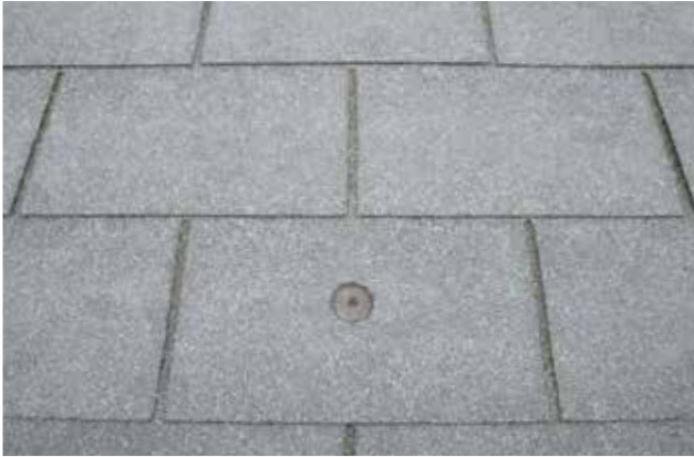
THREE TAB shingle roof
